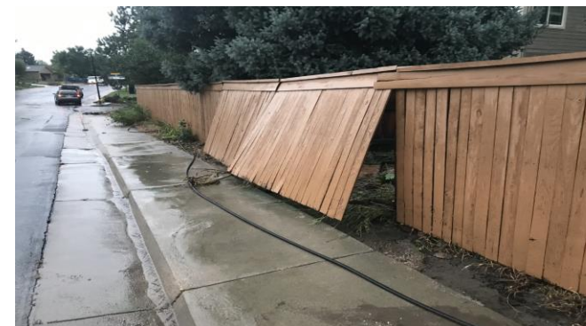
The culvert crossing of Westerly Spring Creek at East Phillips Avenue clogged, resulting in flows overtopping the road damaging private property and an electric transformer in the area
