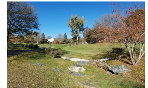
Jamison Tributary conveys flow through open space upstream of the confluence with the Willow Creek East Tributary
